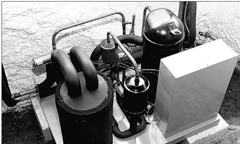
Paul Auerbach of Total Green points out where the outside tubing comes into his basement. It connects with a compressor (below), the heart of the geothermal system. "It takes energy from the ground, and moves it to where it's needed," Auerbach said of the compressor.
