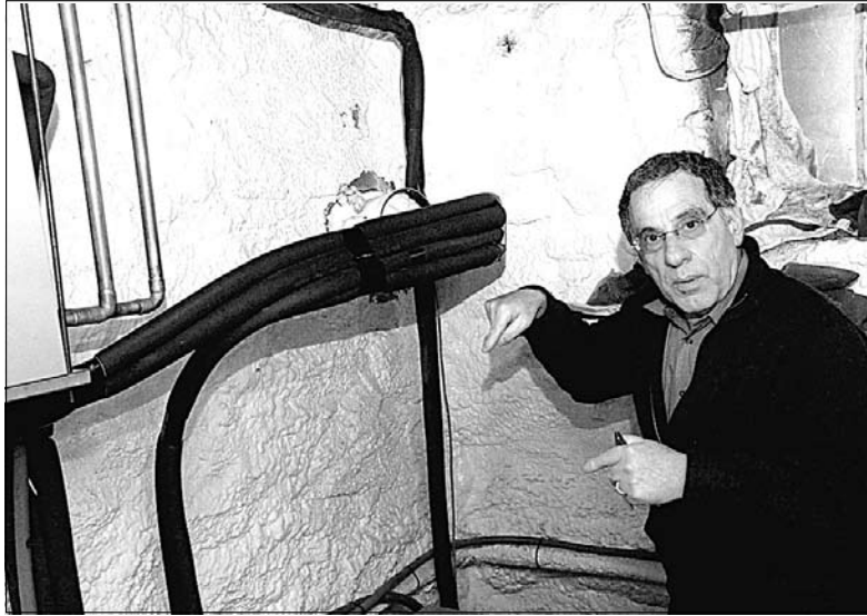
Paul Auerbach of Total Green points out where the outside tubing comes into his basement. It connects with a compressor (below), the heart of the geothermal system. "It takes energy from the ground, and moves it to where it's needed," Auerbach said of the compressor.
